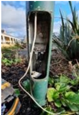
Columns around the café have inappropriate metal clad switch fuses installed
