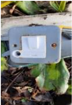
Columns around the café have inappropriate metal clad switch fuses installed
