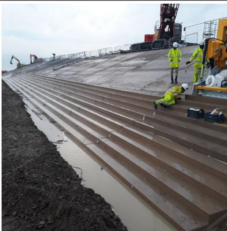
January 2019 – Fairhaven Ch. 900m PCC Stepped Unit Installation
