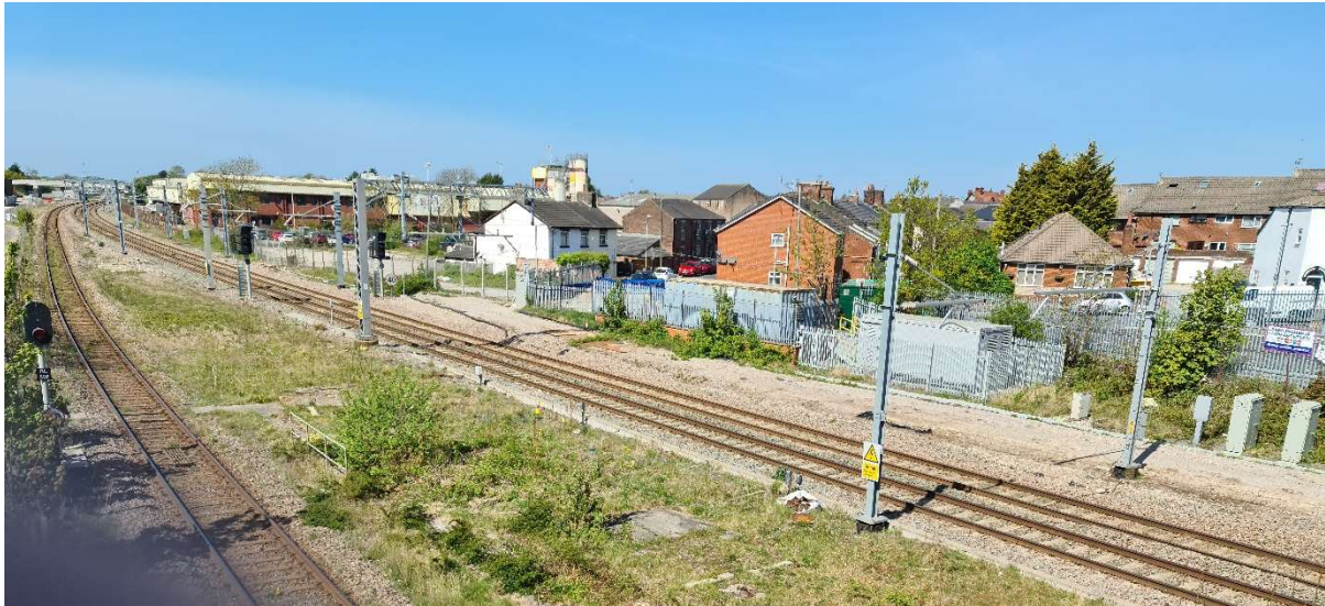
Towards the vehicle entry point
