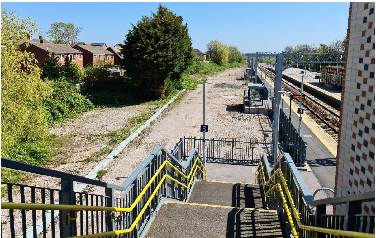
Proposed car park area – generally level with height increase to houses say 1m
