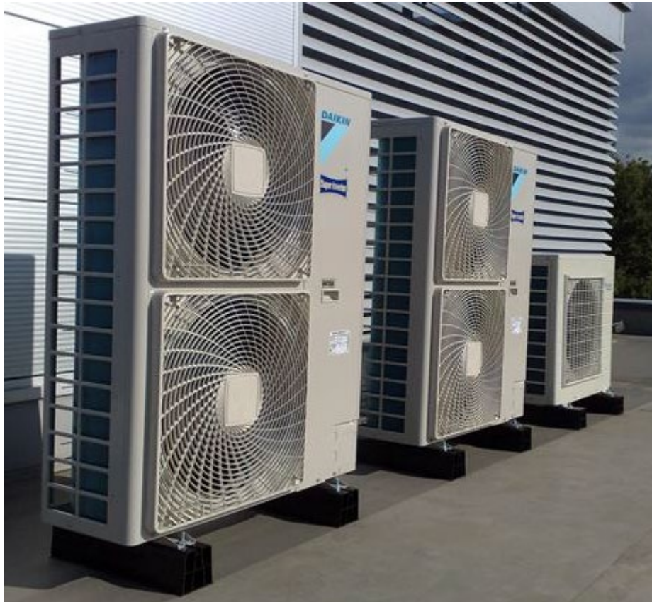
Typical Air-Source Heat Pumps
