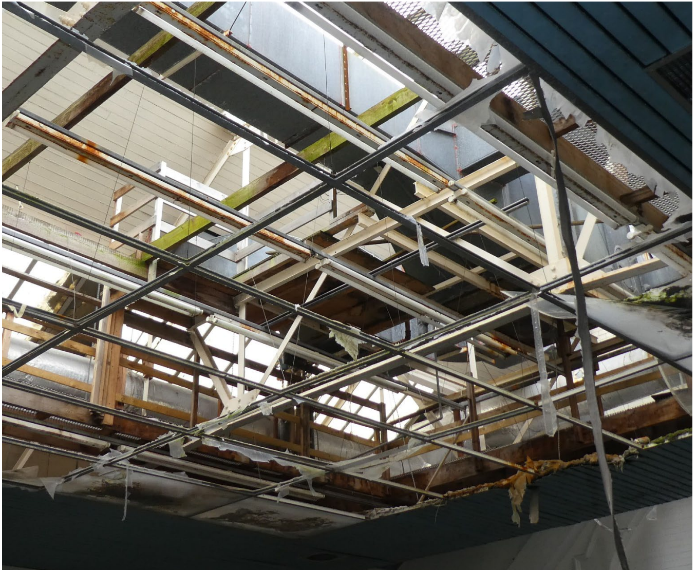
Pool Area AHU
