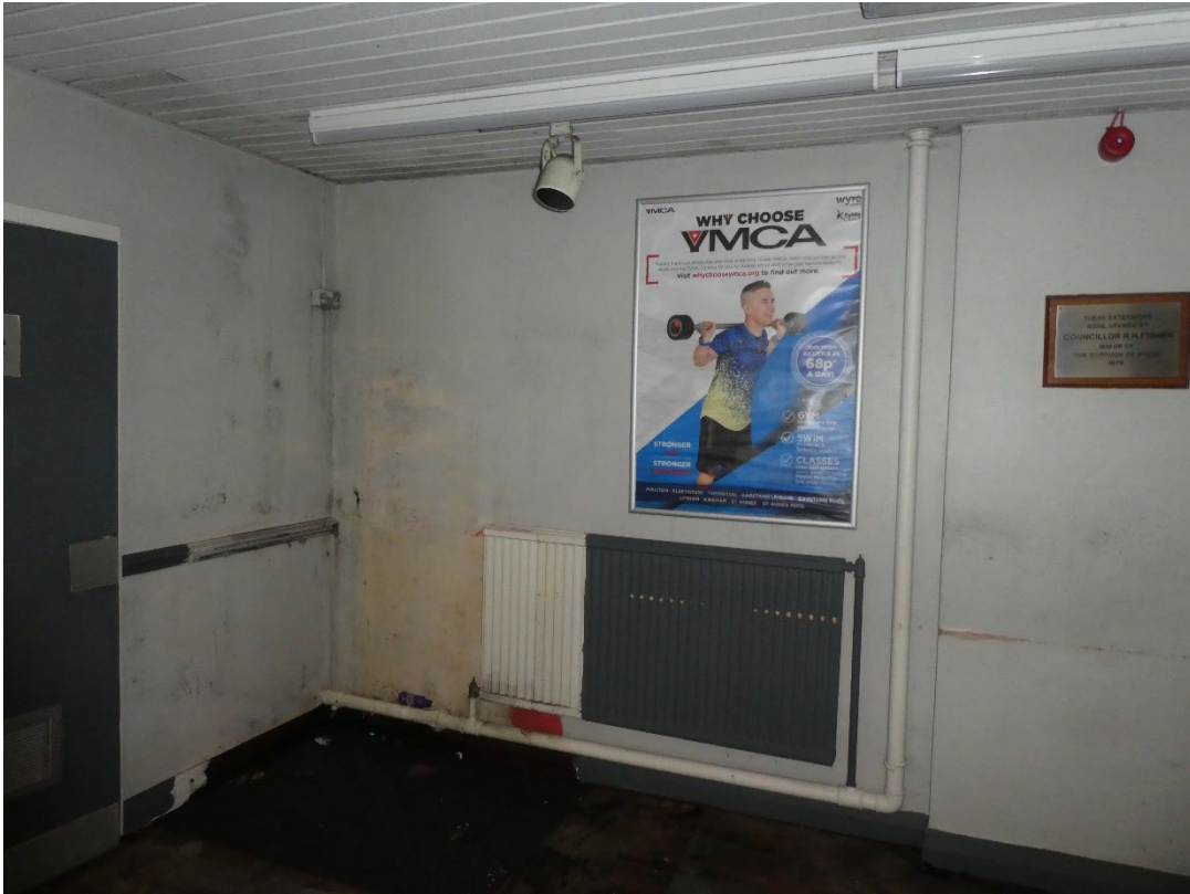
Typical Single-Pipe Heating Distribution
