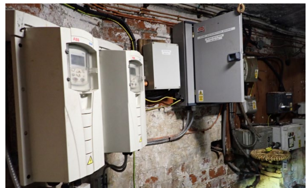
Basement Inverter Controls
