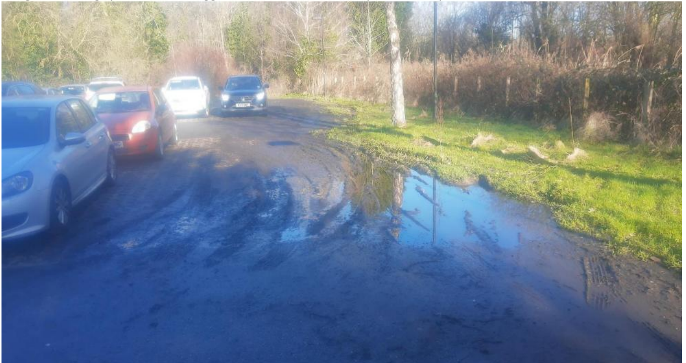
Image 5. Parking spaces near to Liggard Brook which are damp and muddy
