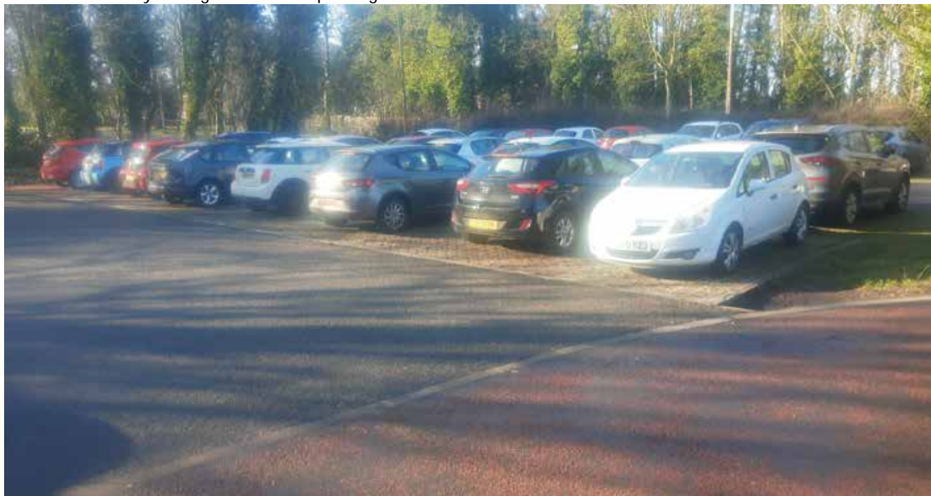
Image 4. Some of the parking spaces within the car park. This shows the difference between the tarmac used for the main roadways and grasscrete for parking areas.
