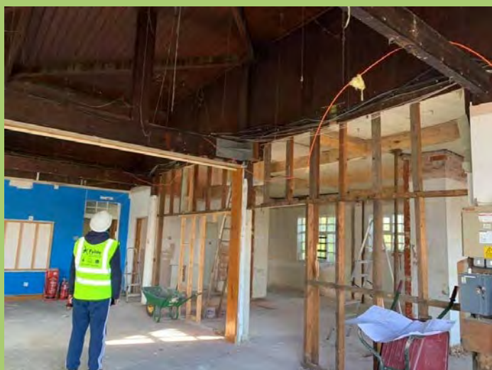
Opening of Pagoda roof void
