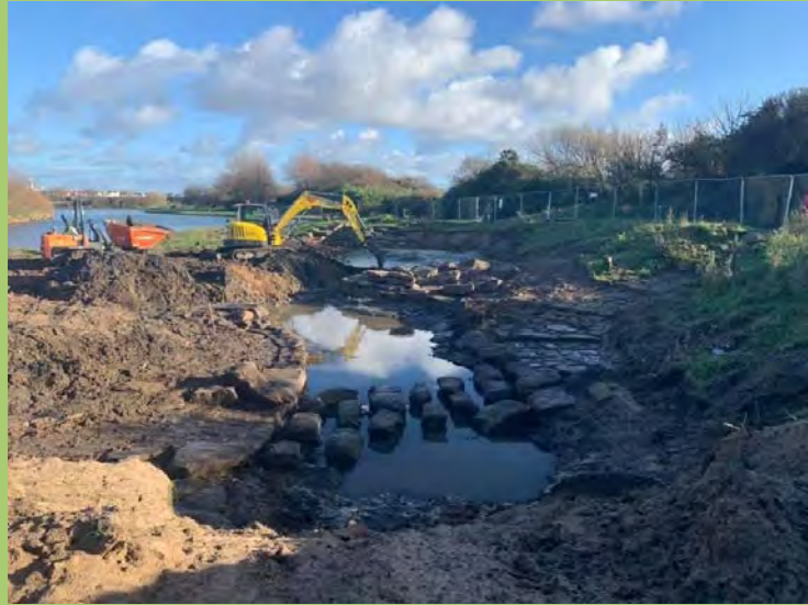
Excavation of Japanese Gardens
