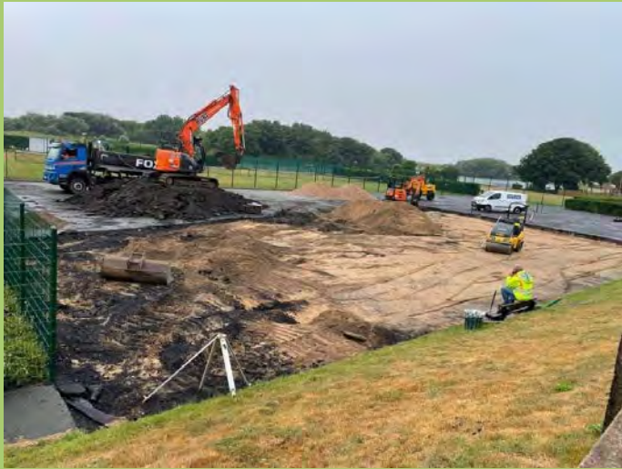
Resurfacing the tennis courts
