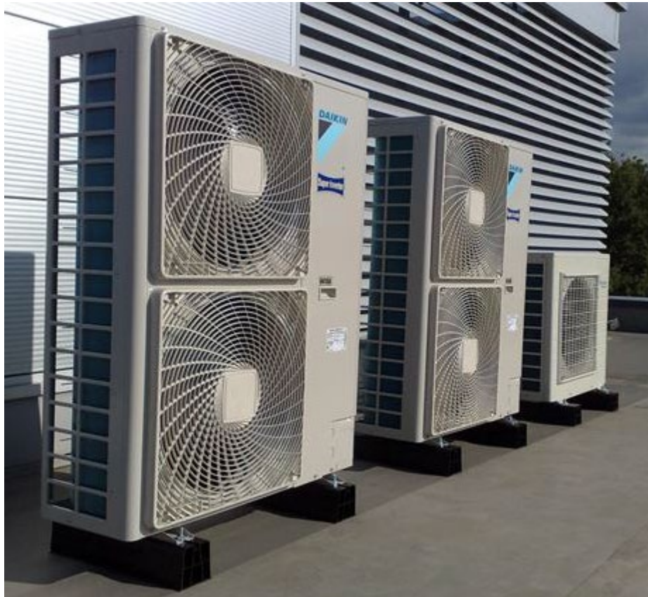
Typical Air-Source Heat Pumps
