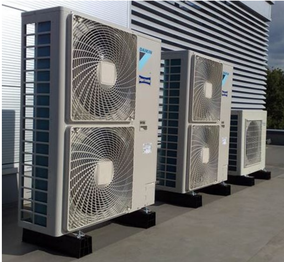
Typical Air-Source Heat Pumps
