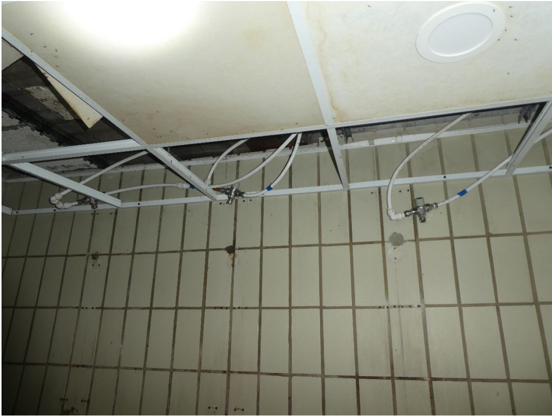
Changing Area Thermostatic Showers (Stripped Out)
