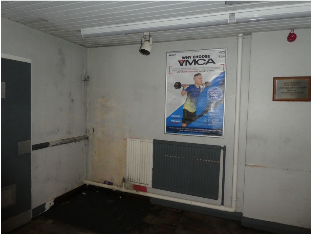
Typical Single-Pipe Heating Distribution
