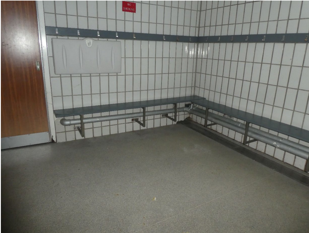
Typical Pipe Heating Coil Under Benches
