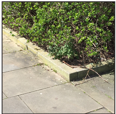
Stone upstand detail to planting beds to match existing on Wood Street and Park Road
