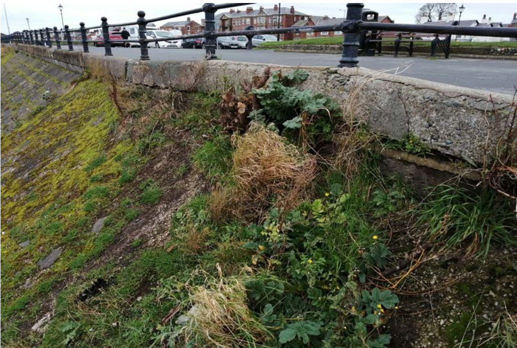
Image 2 - Existing plinth wall being undermined by vegetation
