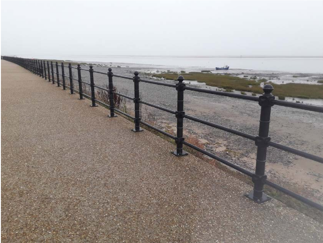
Image 3 - Proposed replacement detail – as delivered west of Church Scar. Note the old stone revetment has been retained in this area.
