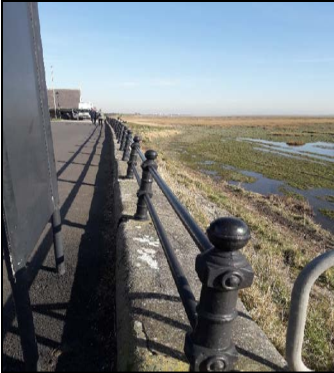
Image 1 - Existing plinth wall which is leaning seaward adjacent the windmill.
